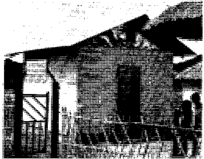
Figure 23. Simple naturally-ventilated stores. A -- Timber, 20 TM capacity (CIP, Huancayo, Peru). B -- Mud-brick or concrete block, 15 TM capacity (CIP-PCARR-MSAC, Baguio, Philippines).
