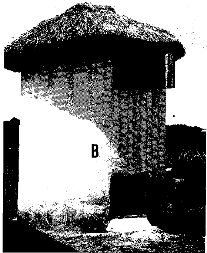
Figure 21. Simple, small rustic stores with outside painted white. A -- Timber construction, 1.5 TM capacity (CIP, Huancayo, Peru). B -- Lath and plaster and mud brick construction, 2 TM capacity (Mountain State Agricultural College, Baguio, Philippines).
