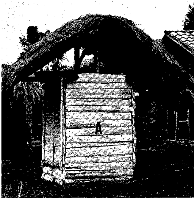
Figure 21. Simple, small rustic stores with outside painted white. A -- Timber construction, 1.5 TM capacity (CIP, Huancayo, Peru). B -- Lath and plaster and mud brick construction, 2 TM capacity (Mountain State Agricultural College, Baguio, Philippines).
