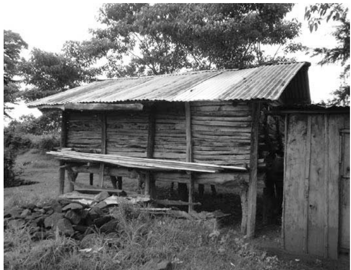
Figure 12a: Maize store in Kenya converted into diffused light store. (outside view)
