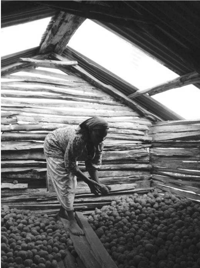
Figure 12b: Maize store in Kenya converted into diffused light store. Note that shelves are still missing (inside view)
