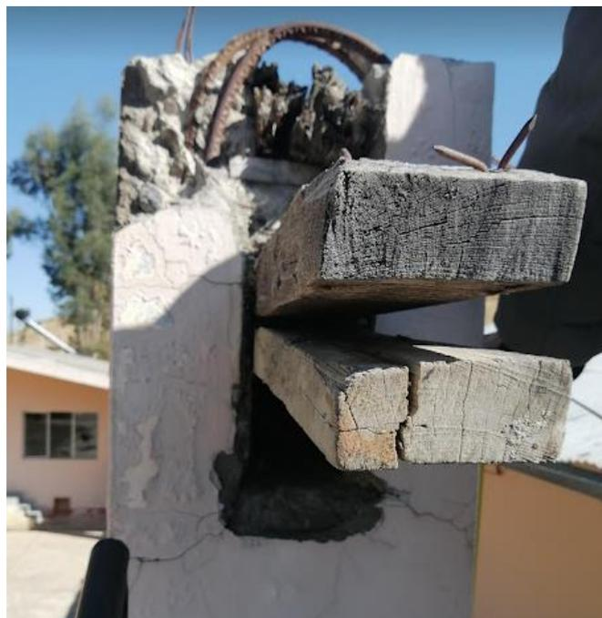
**COLUMNA EXISTENTE DONDE SE REALIZARÁ CORTE**
