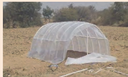
Fig. A5.14. Netting laid over frame with 20 cm allowance at ground level, and 10 cm at front and back
